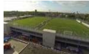
Rooftop Soccer with water retention
